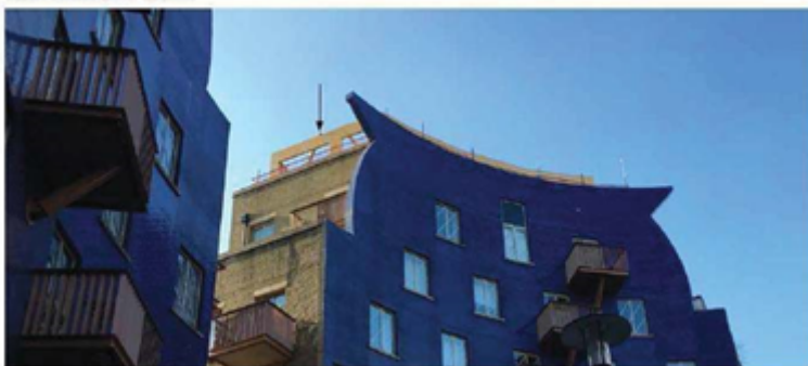
Site progress under NMA 15/AP/0060
