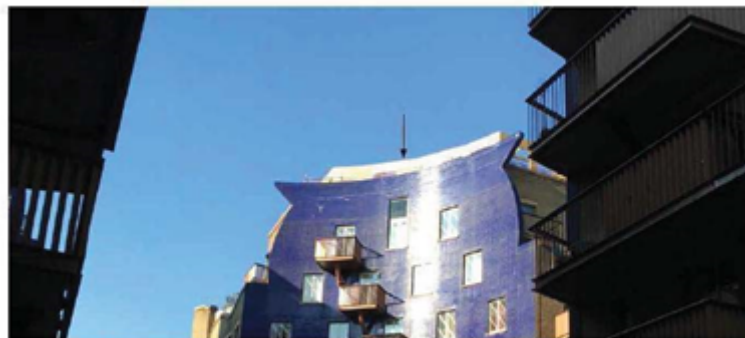
Site progress under NMA 15/AP/0060
