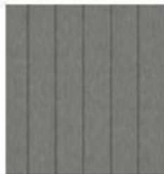
2. Vertical standing seam zinc cladding - adhering to the language of a mansard roof
